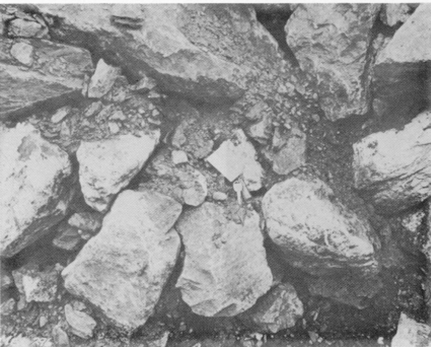
Figure 12-19. Photographs of sound rockfill, New Melones Dam test fill inspection trench
