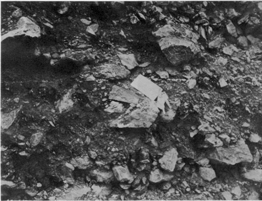
Figure 12-20. Photographs of rockfill containing appreciable fines, New Melones Dam test fill inspection trench
