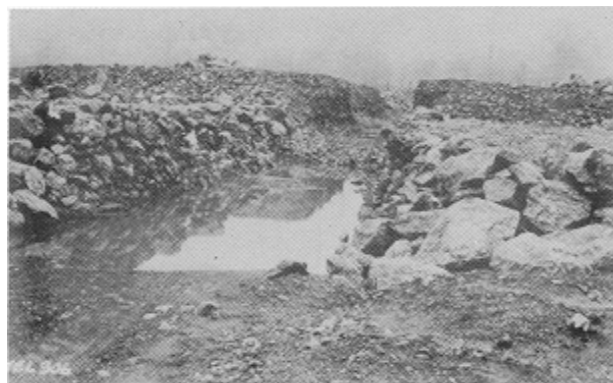
Figure 11-6. Inspection trench through the New Melones Dam test fill
